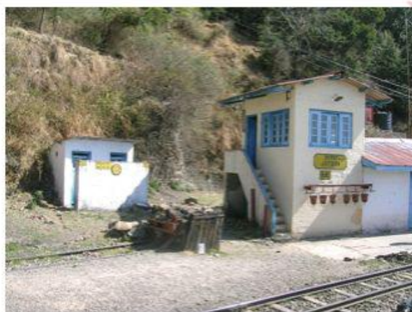
Jutogh signal box and station conveniences.
