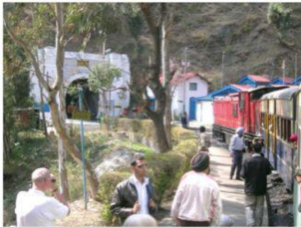
The rather fine entrance to Barog Tunnel.
