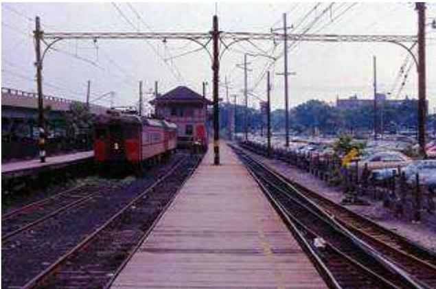
The second image is at Gary, Indiana on the South Shore Line (Chicago, South Shore & South Bend Railroad) and allows over wide freight cars to pass through the station. As the South Shore Line once operated some of the largest electric locomotives in the USA, the General Electric 2-D+D-2 "Little Joe" locomotives, the extra clearance was absolutely essential.
