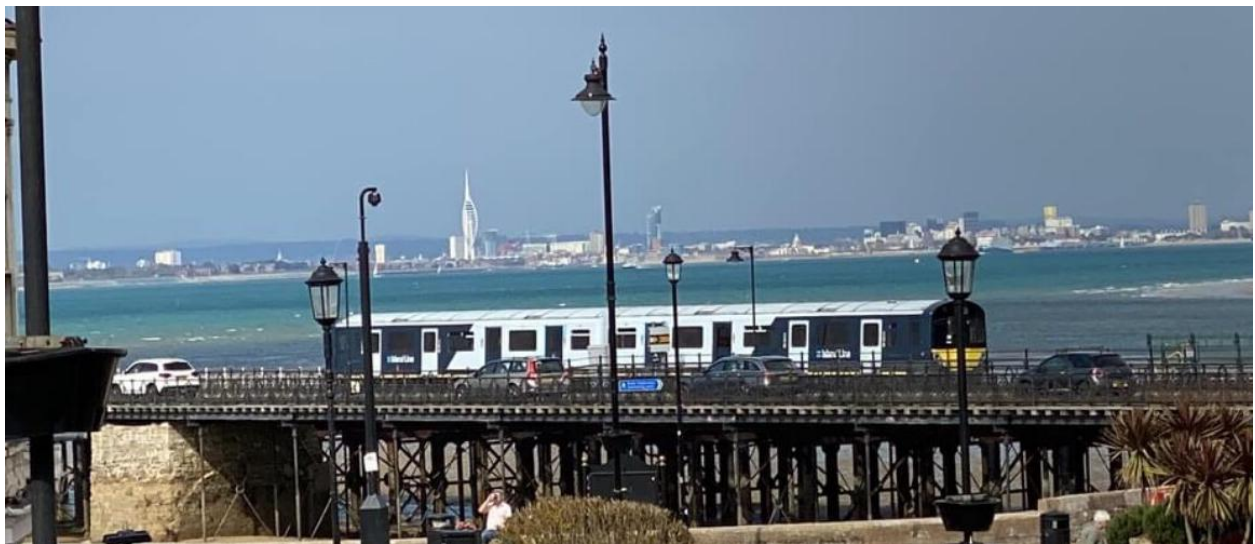
Above - class 484 on Ryde Pier.
