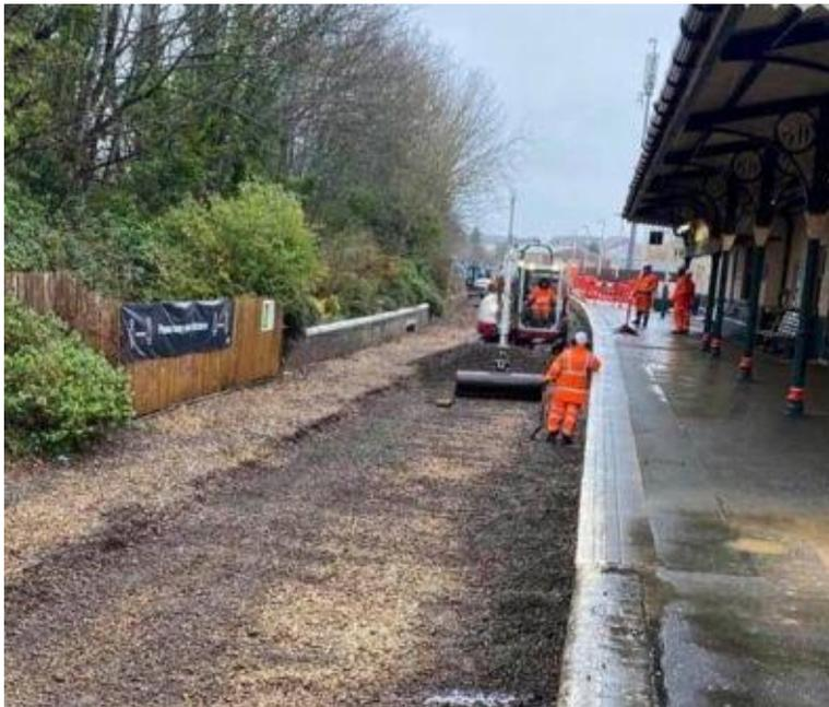
Additional works will be involved to correct for the platform height, as the Class 484 rides substantially higher than the outgoing Class 483. Work on lowering tracks is seen in progress at Shanklin (photo by Mark Herbert) whilst at Smallbrook Junction, Lake and Sandown the platforms have been raised.
