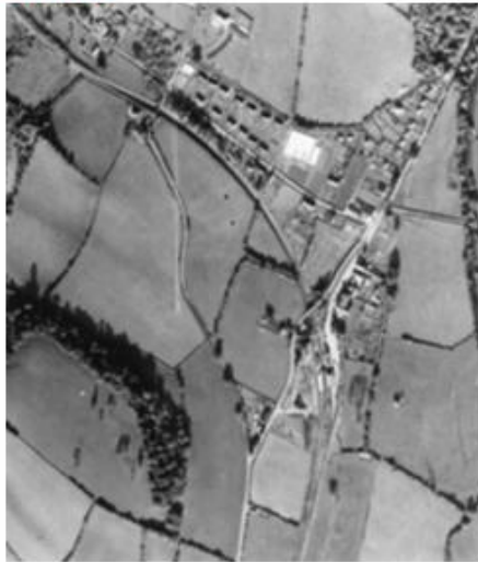
Dulverton station – RAF 1952
