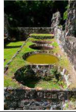
Boiling room with series of kettles, "refined" sugar is ladled from one to the next one to improve clarity
